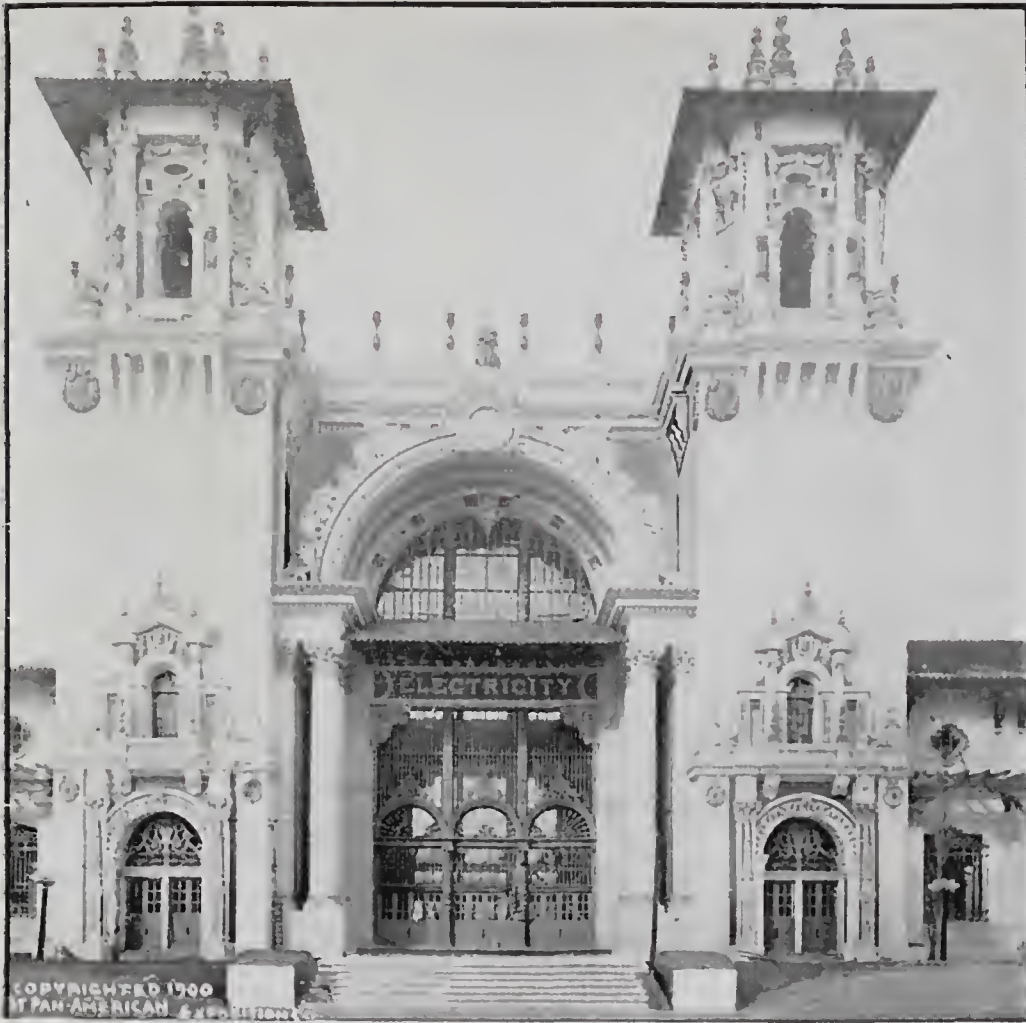
SOUTHERN ENTRANCE, ELECTRICITY BUILDING.
